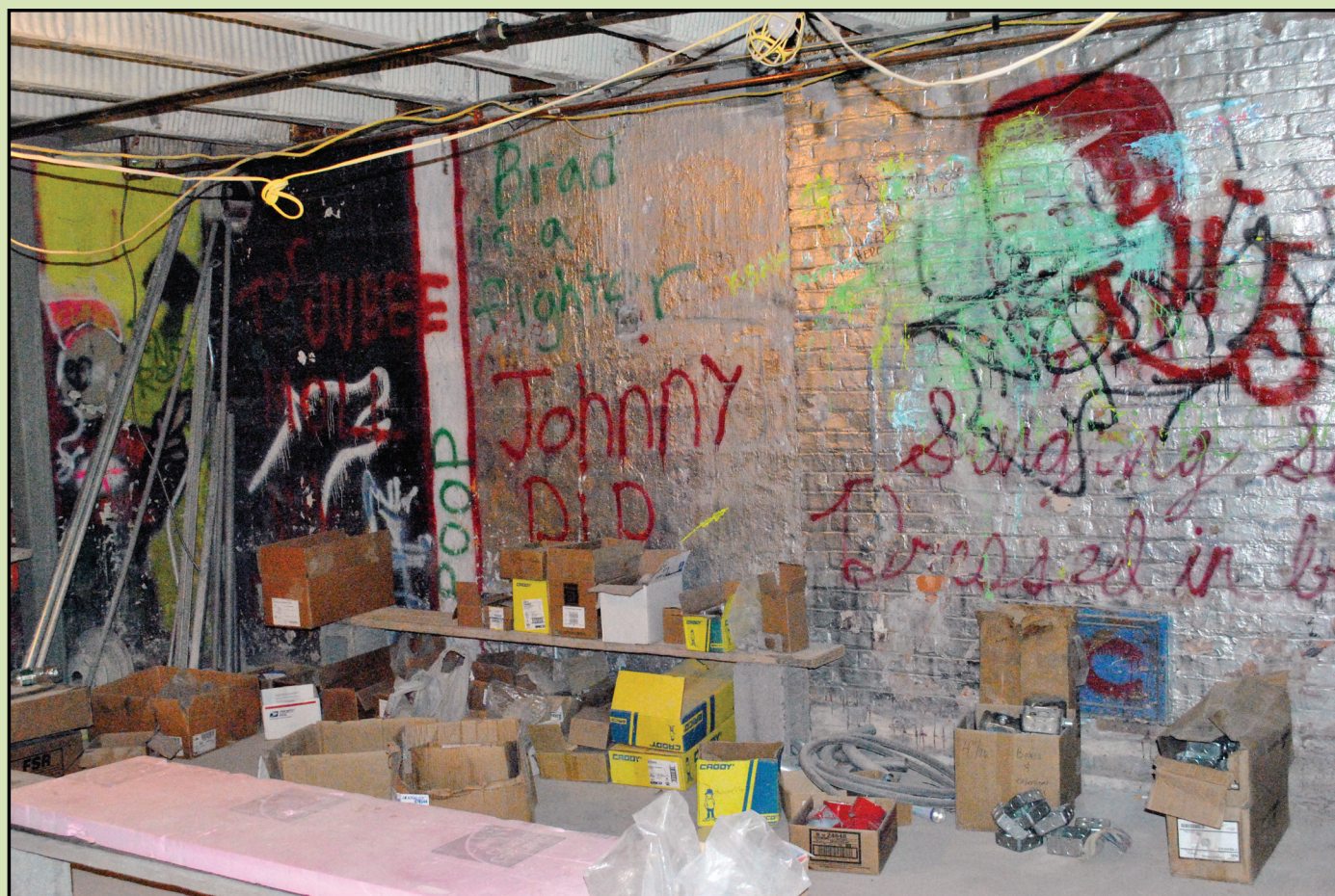
The basement of ELS, shown here, will continue to serve as a space for parties. New additions will include a coat room, a kitchenette and a small stage at the back to accommodate performance groups such as student bands. The graffiti that covers the walls, however, will be removed.
